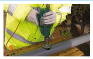
2. Mark out the area covered by the saddle on the pipe.
