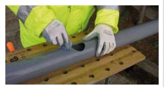
4. Feed on to pipe two worm drive (Jubilee) clips which will clamp the saddle during fitting. These should be placed either side of the socket on the saddles. Apply cement to pipe area and saddle. It is important to apply cement quickly.
