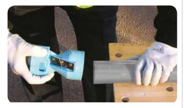
Mark the pipe a known distance from the end and clear of the area to be cleaned. This mark should be used to confirm full insertion of pipe into socket of fitting.
